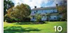
PRESIDENT'S HALL Alumni Relations/Advancement College Relations Executive Offices Office of the President
